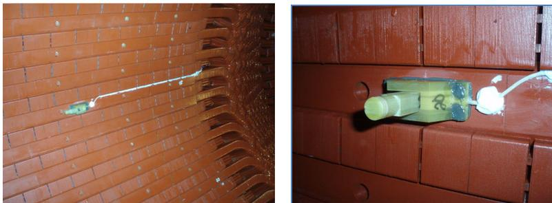
**Figure 12:** *Installation of air gap sensor at stator winding slot wedge*
