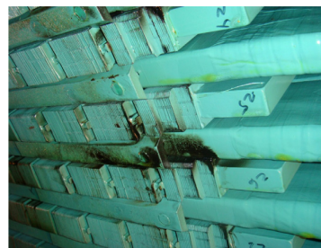
Fig 6: Photograph of a 150 MVA hydrogen-cooled turbine generator that had extensive greasing at the slot exits due to loose bars in the slot. The side packing was also abraded. The associated PD data is shown in Fig. 5.
