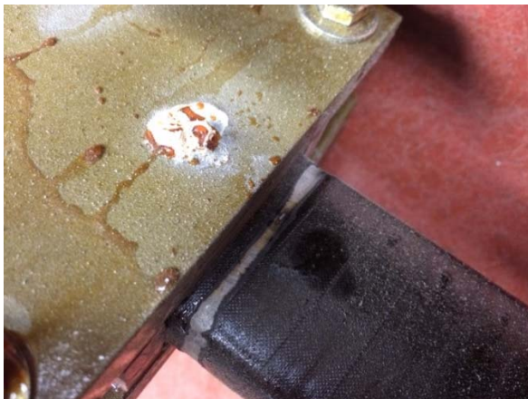
Fig 3. Damage simulation on conducting armour of a VPI'd coil rated 13.8 kV
