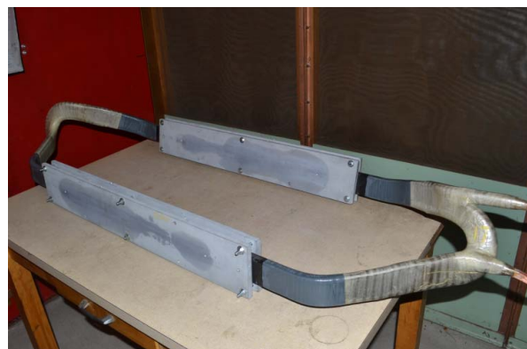
Fig 3: PD test setup without insulating blocks.
