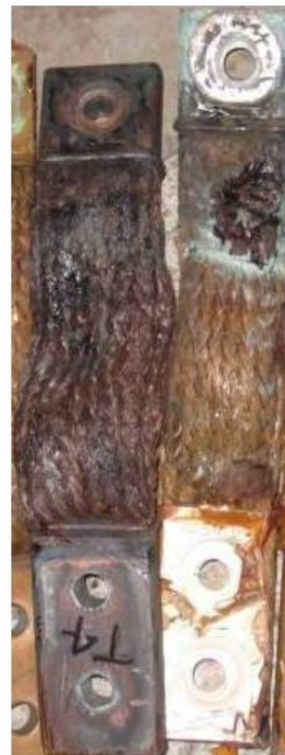
Figure 7: Overheated motor terminal leads
