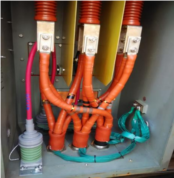
Fig. 6 Installation of 3 PD sensors (behind the power cables) and a voltage divider (in the foreground) in the terminal box of an IFM.
