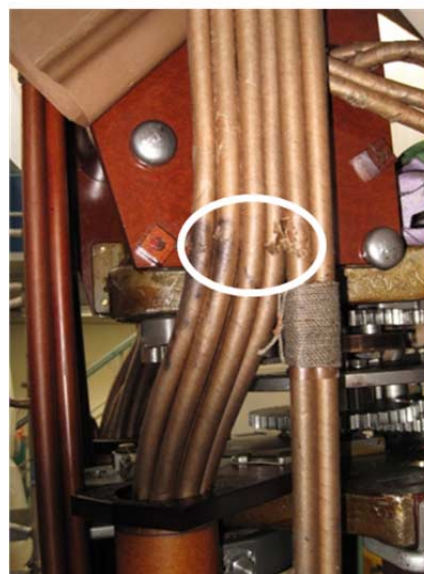
Figure 11 Deteriorated paper insulation on leads at the tap changer.
